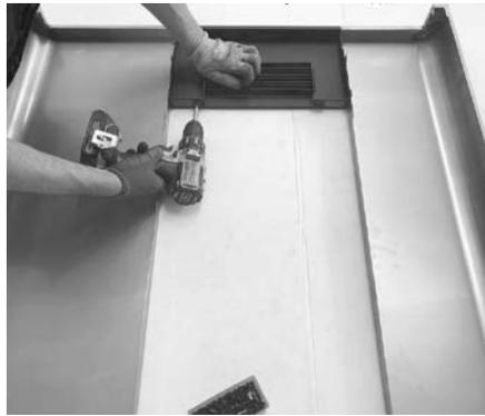
**Fig. 43 - Secure the grate**
