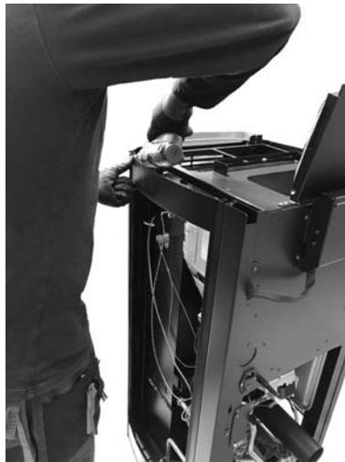
*Fig. 52 - Remove the compensator*
