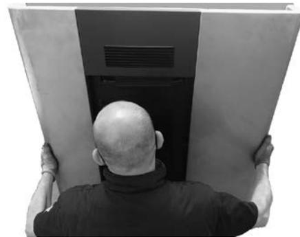
**Fig. 46 - Position the frame**
