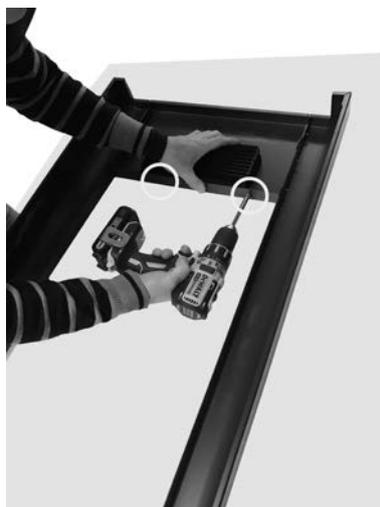
Fig. 23 - Secure the grate
