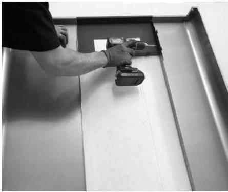
**Fig. 42 - Secure the strut**
