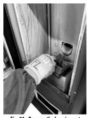
Fig. 91 - Remove the burning pot
