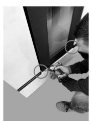
Fig. 44 - Fix lower panel
