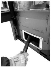
Fig. 95 - Vacuum out the ash
