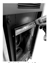
Fig. 96 - Remove the deflector
