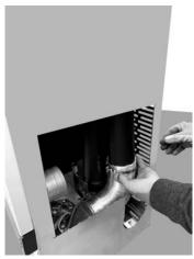
Fig. 83 - Connect the pipes
