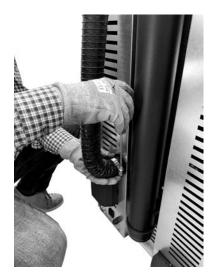
Fig. 56 - Insert combustion air pipe
